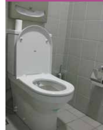
Toilet installed in the basement
