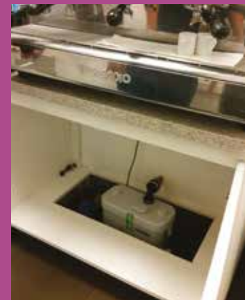
SANISPEED® pump installed to remove kitchen waste water
