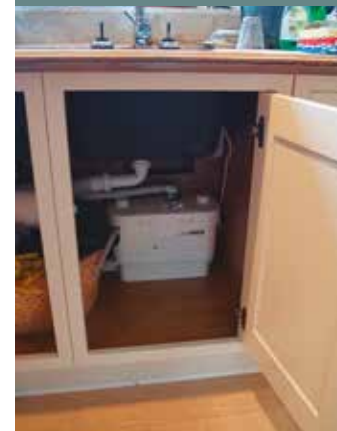
SANISPEED® pump discreetly installed under the sink
