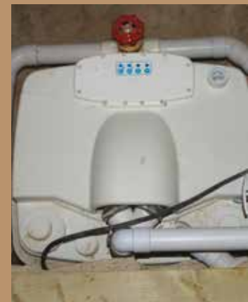
SANICUBIC® 2 Pro lift station installed in the basement
