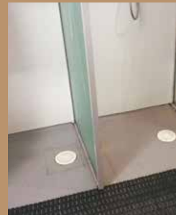
Collective bathroom located in the basement
