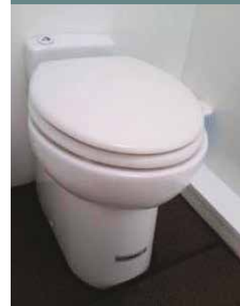
SANICOMPACT® Pro installed in order to drain waste water to the tank
