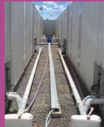
SANIBEST® Pro removes waste water to a holding tank
