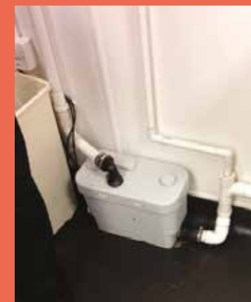
SANISPEED® pump installed in the basement
