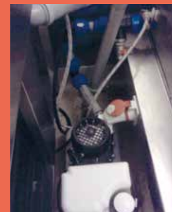
SANICOM® 1 lifting pump installed
