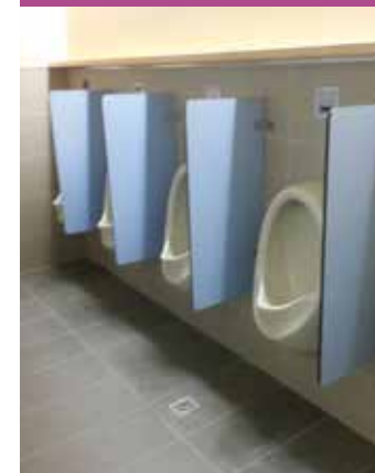
Toilets installed for factory staff
