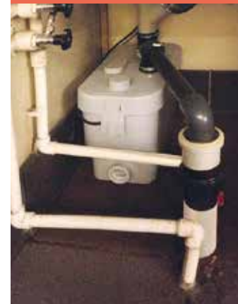
SANISPEED® pump installed under the sink
