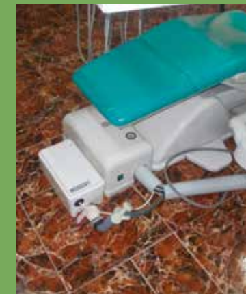
SANISHOWER® pumps installed to drain waste water from sinks
