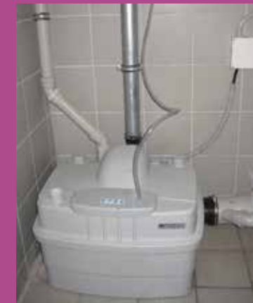
SANICUBIC® 2 Pro lifting station installed in the basement to remove waste water
