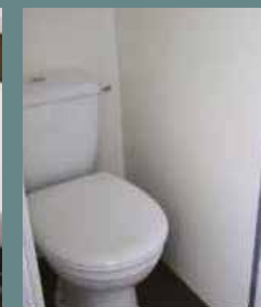
Toilet and shower installed
