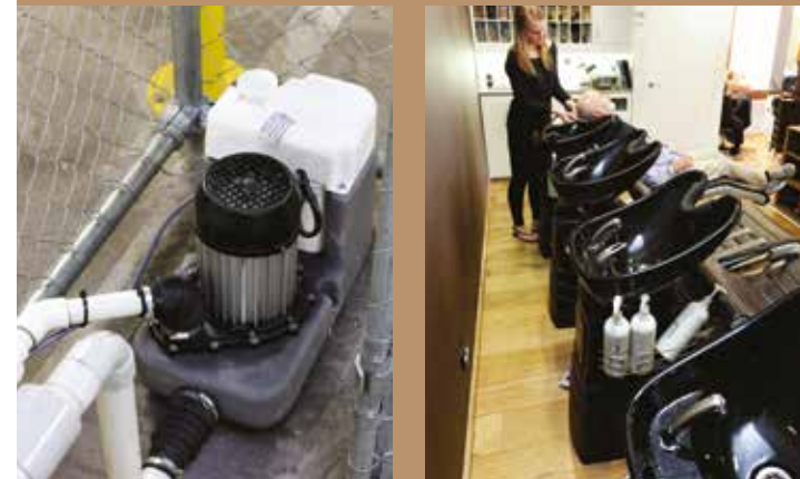
SANICOM® 1 installed near the hairdressing salon
